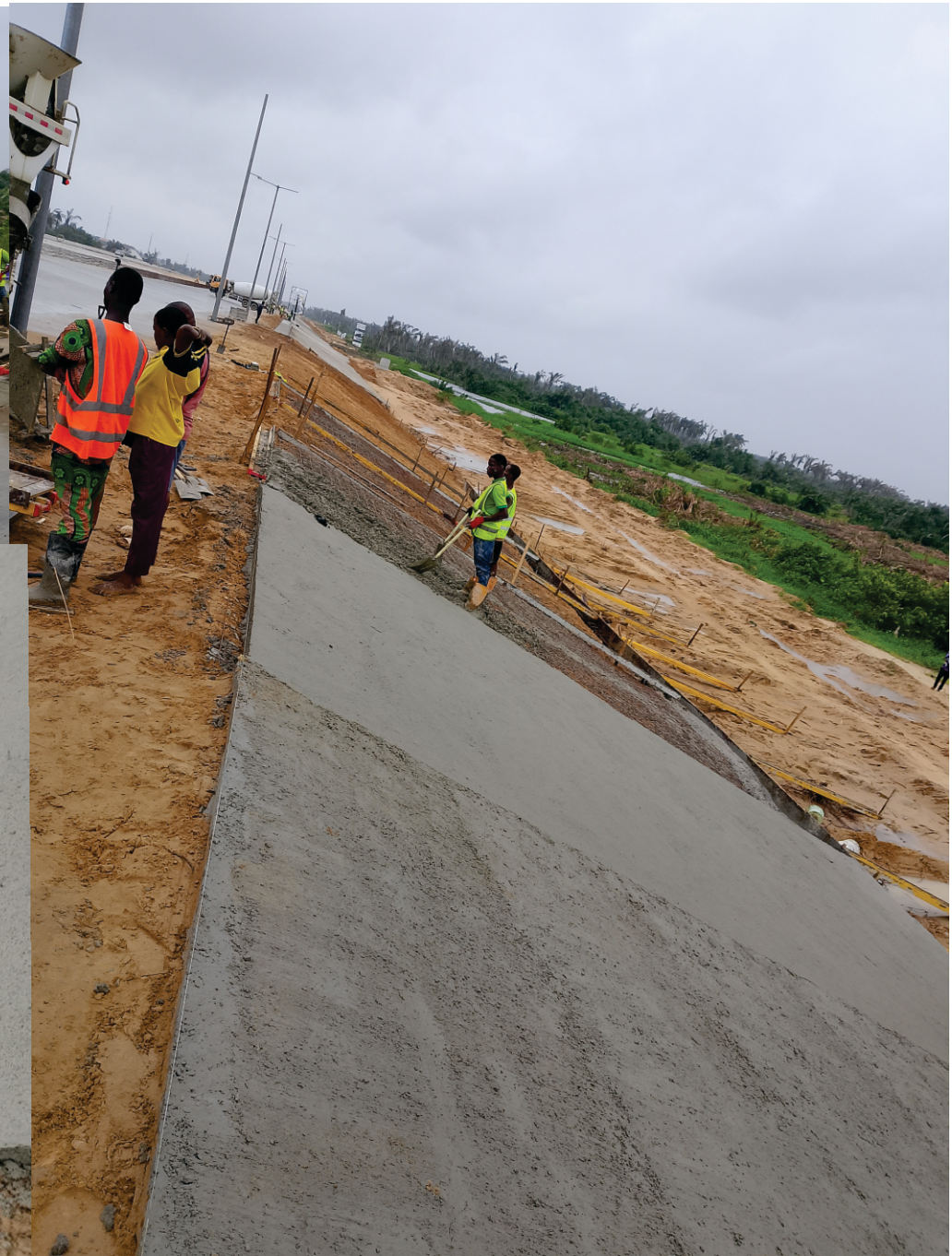
REENFOCE CONCRETE SLOPE PROTECTION @ HITECH CONSTRUCTION BY JOHNSONWEST
