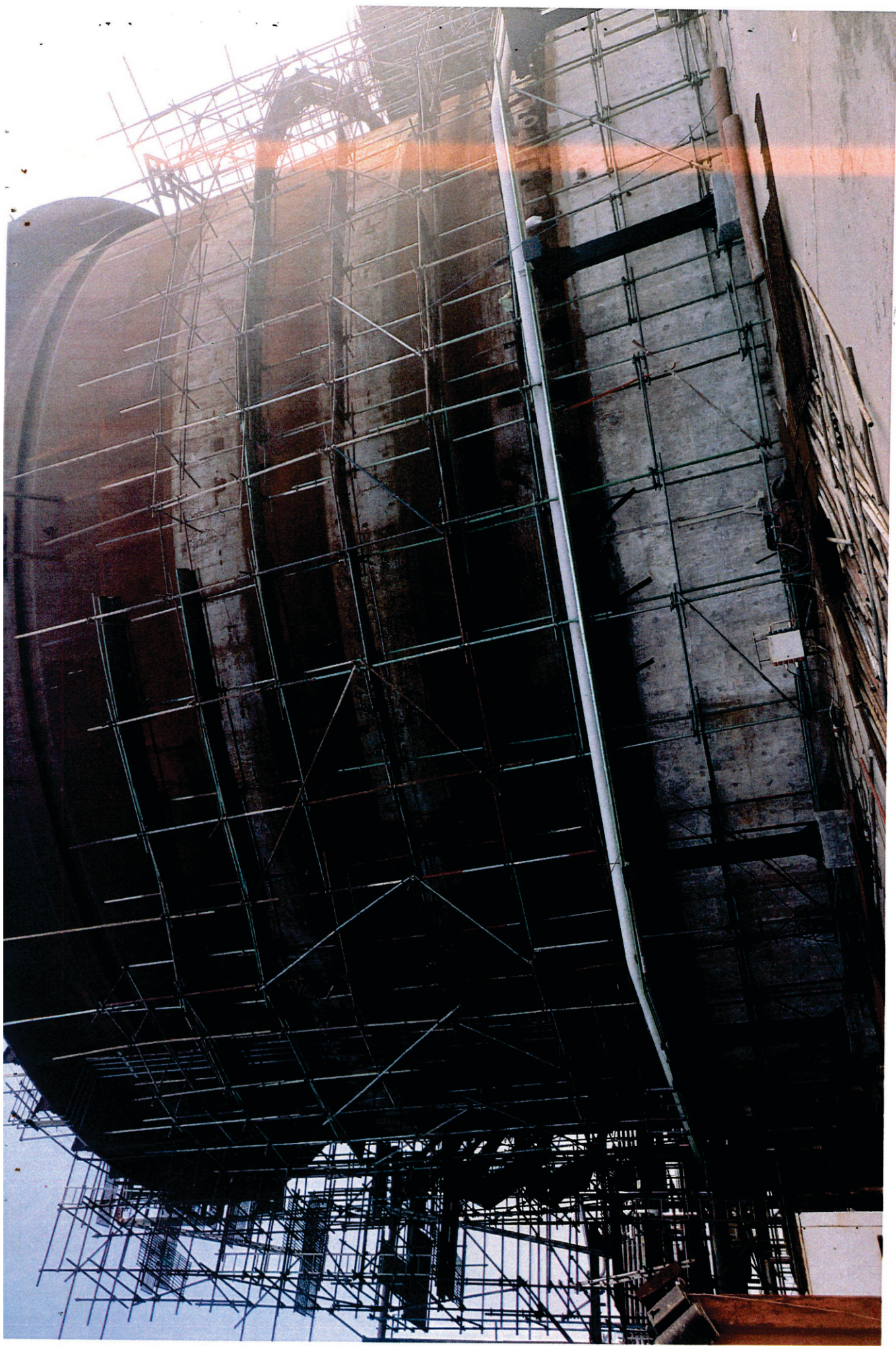
ongoing scaffolding Work at Tank 2 SRU Department Dangote Refinery LFTz Ibeju-Lekki Lagos State
