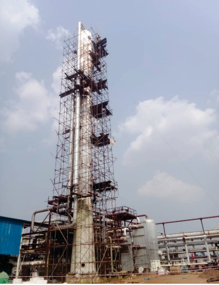
45MTS HEIGHT VESSEL SCAFFOLD ERECTED @ GAS PROCESSING PLANT @ OGBEANI COMMUNITY, (GPP I & ii) KWALE, DELTA STATE
