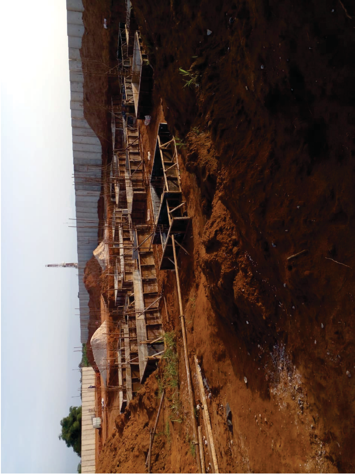
BUILDING A3 FORM WORK AND REINFORCEMENT ARRANGEMENTS. AT SEEPCO COMPANY IMO STATE
