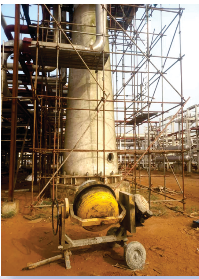
45MTS HEIGHT VESSEL SCAFFOLD ERECTED @ GAS PROCESSING PLANT @ OGBEANI COMMUNITY, (GPP I & ii) KWALE, DELTA STATE
