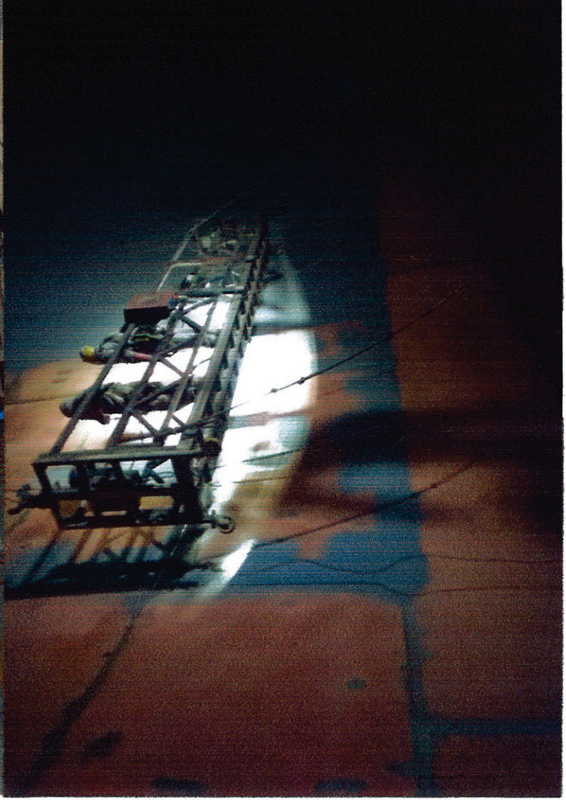
Blasting & Painting of 91 dial Tank at Dome Tank @ chemie-tech Construction Company @ dangote Refinery Oil company Ibeju-Lagos state( confined Space Blasting & painting With Gandolla)
