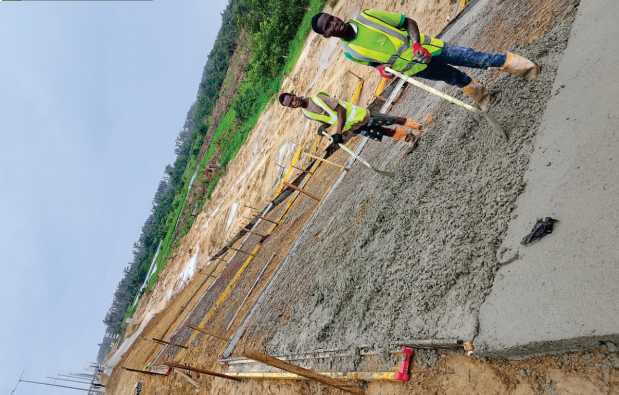
REENFOCE CONCRETE SLOPE PROTECTION @ HITECH CONSTRUCTION BY JOHNSONWEST
